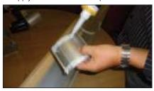
**3** Locate clip ensuring that the clip MUST clip into both sides of the gutters.
